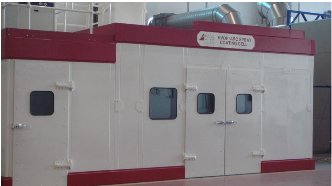
Picture 16: Bay 2 - Automated ABB Robotic Spray System incorporating Praxair JP 8000 HP/ HVOF & 8853 ARC Spray Coating Cell
