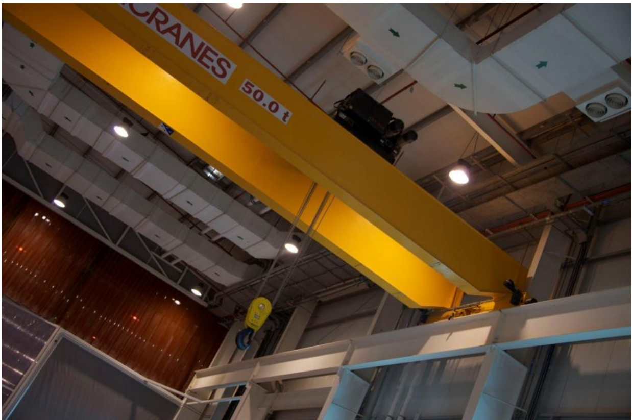
Picture 6: Bay 1 -4 – Dual Carriage 50T overhead crane in each bay
