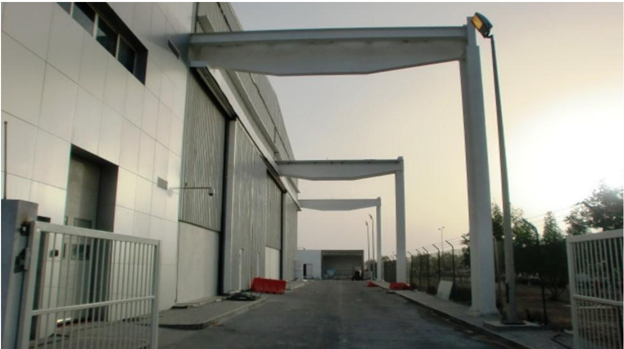
Picture 4: Workshop Delivery Entrance – 2x50T Overhead Cranes can come out of the workshop and lift material from the delivery truck to minimise handling
