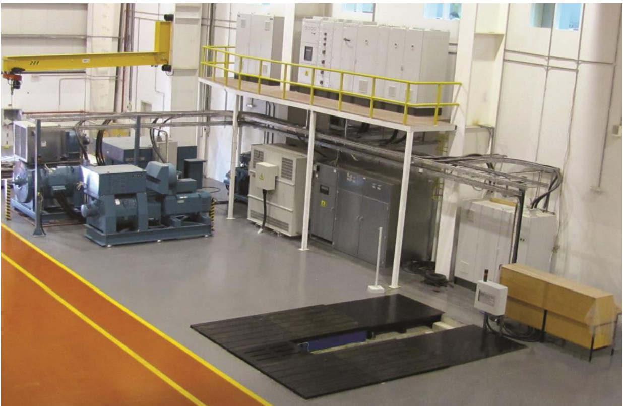
Picture 18: Bay 4 –Electrical Test Station
