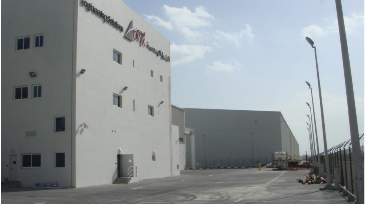
Picture 3: Rear of Facility - Laydown Area
