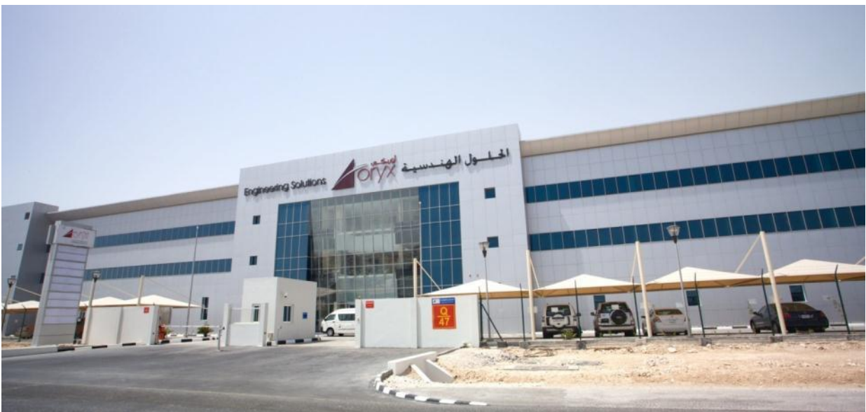
Picture 2: Main Front Entrance of Facility
